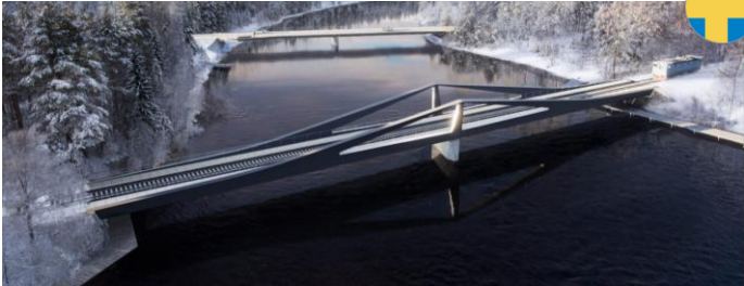
Bridge project, Oxberg
